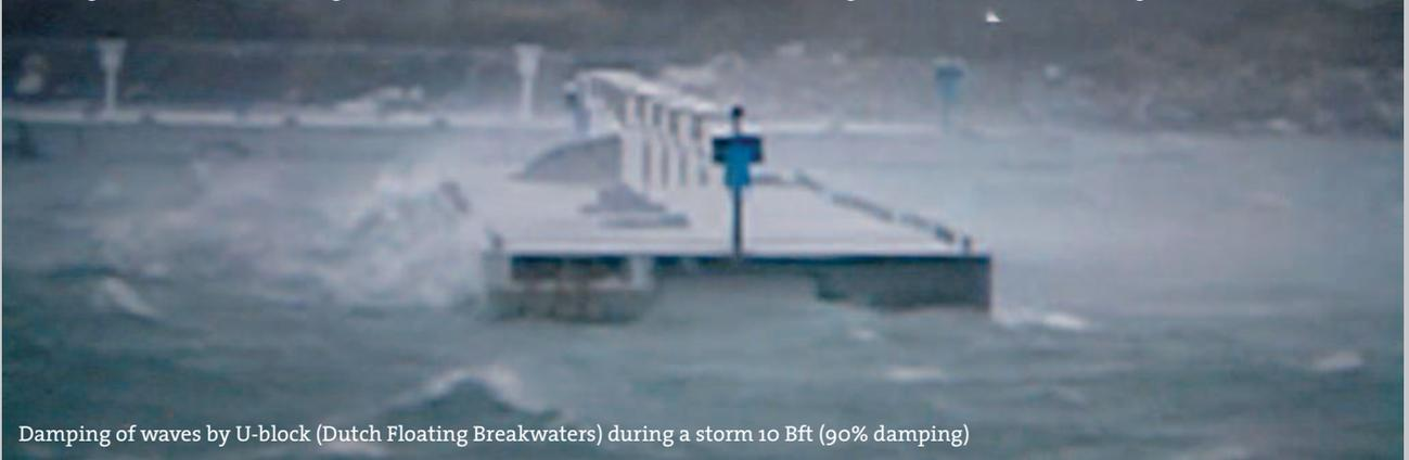
Damping of waves by U-block (Dutch Floating Breakwaters) during a storm 10 Bft (90% damping)
